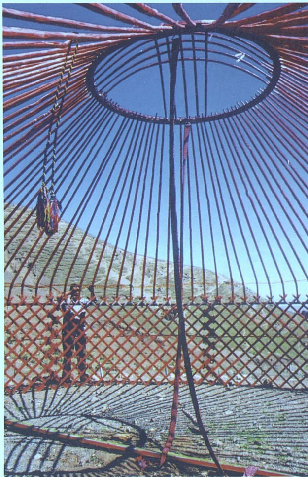
Үй тігу 搭建毡房 The frame work of a circular roof yurt
